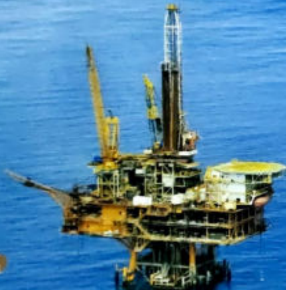
A state-of-the-art rig mounted platform RS-12 for expeditious production
